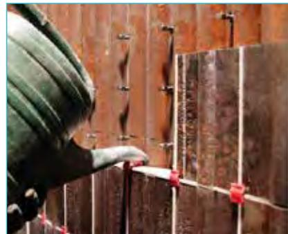
Figure 4: Back-filling of the liner/spacer stabilised SiC tile wall
