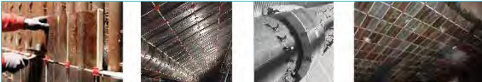
Figure 1: The system can be used even in geometrically difficult areas such as corners, curved tube sections and on collectors (headers); in the past this could only be done with (SiC) castables and (SiC) ramming materials
