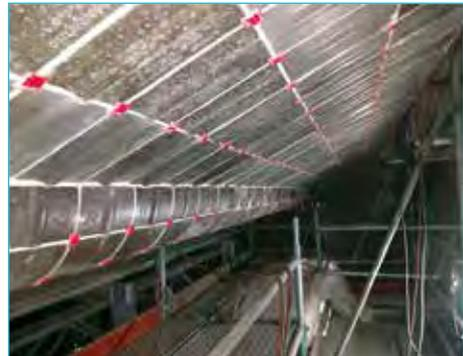
Figure 6: Boiler tile system mounted on the prism membrane wall
