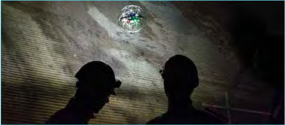
Figure 25: Boiler inspection with a JuSpect drone
