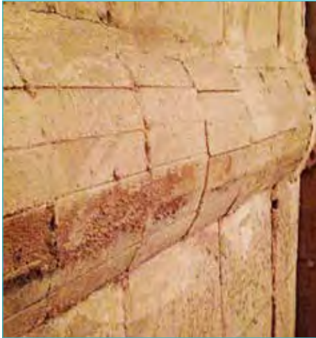
Figure 15: In operation since 2014 maintenance-free
