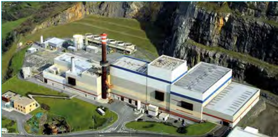
Figure 9: Area of WtE integrated in Artigas-Arraiz Special Plan in Bilbao
