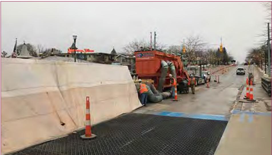
Figure 1: Draw bridge maintenance being performed, employing a containment enclosure and a large mobile dust collector
