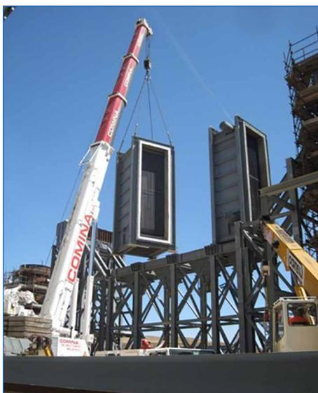
Figure 9: Typical modular boiler assembly
