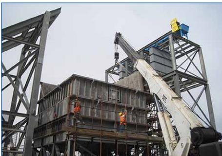
Figure 8: Typical ASGC reactor panel assembly
