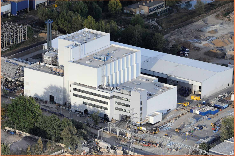
Figure 5: The EfW plant in the Polish city of Poznan was handed over to the client in 2017
