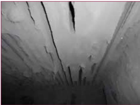
Figure 11: Before installing infrasound cleaning: severe fouling in the lower part of the ECO after 5 months
