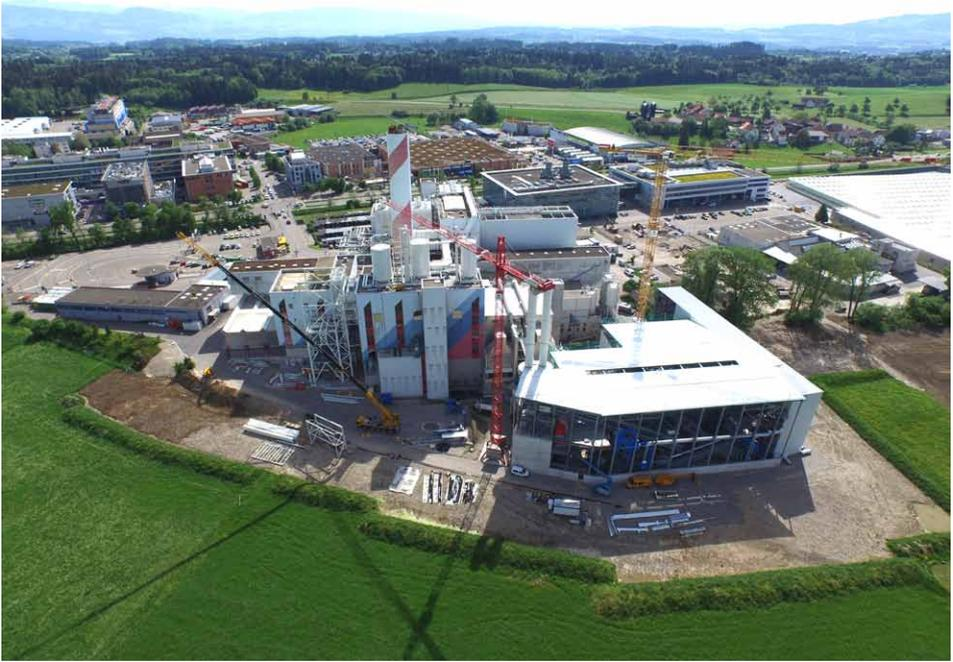
Figure 3: Construction site of the new processing plant for dry bottom ash in Hinwil, Switzerland, adjacent to the municipal waste incineration plant KEZO
