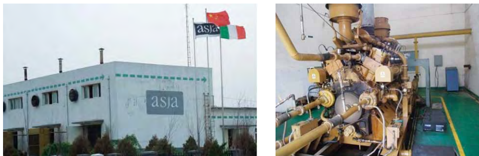
Figure 2: Three of six cogeneration of CHP units of Shenyang Laochuchong Landfill 3,000 tons/day, grid connection operated as CDM project by Asja, Italy
