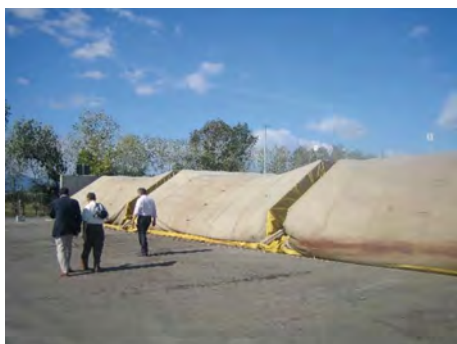
Figure 1: MBT and landfill, one of the first plants in Italy using side walls and GORE Cover starting operation with 35,000 tpy; Handling Cover: manually
