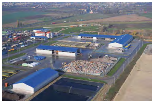
Figure 4: 160,000 tpy, Recycling Park, MSW, Started operation in 2009, Production of high quality compost from separate collection, RDF for the cement industry, Stabilized organic towards landfill; Handling Cover: Winder on the push wall
