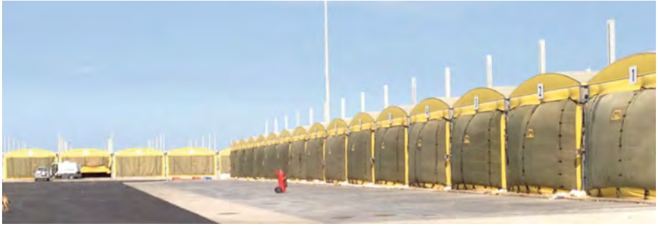
Figure 14: Intensive rot – stabilization, drying of < 65 mm fraction
