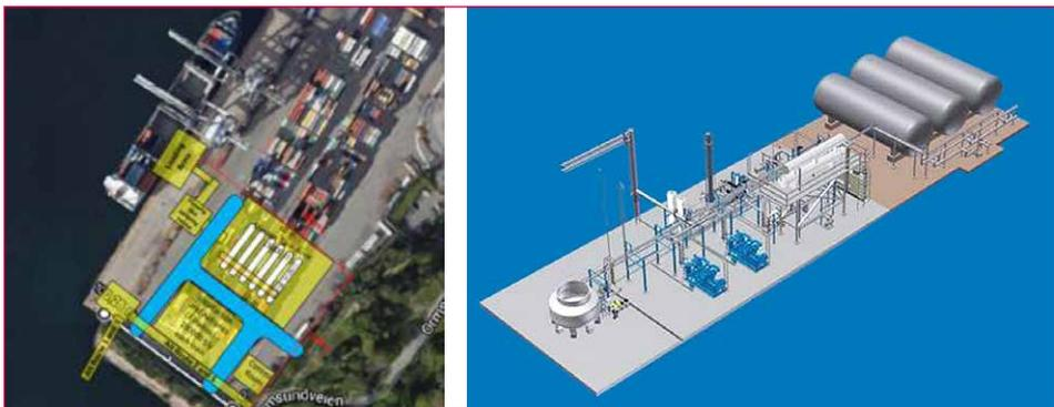
Figure 3: View of possible location at Ormsund Quay with intermediate (left) and typical small-scale CO<sub>2</sub> storage facility (right)
